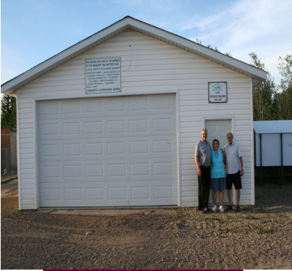
Storage shed after upgrades
